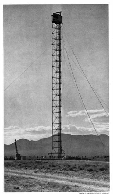
Bomb, resting in cab at top of 300-foot tower, normally disintegrates the entire structure. Disarmament team had to climb ladder to cab, remove crucial wires
